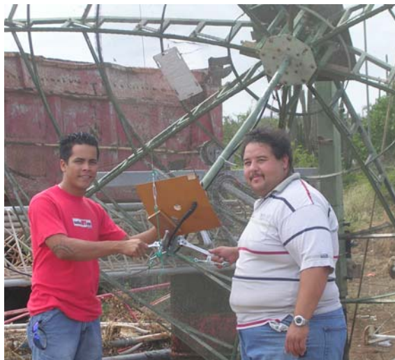
P43L and friend installing 432 MHz feed
