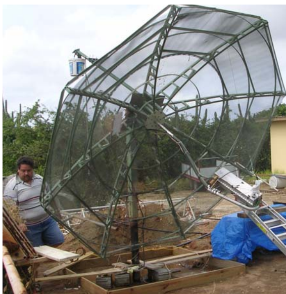
Mounting and installing dish
